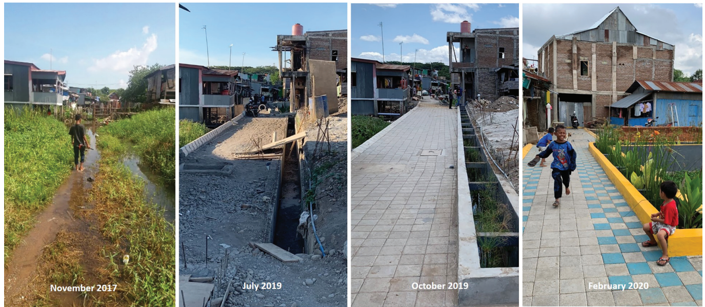
Fig 1 | Water sensitive slum upgrading interventions providing flood-free and contamination-free access to dwellings with a sewage network and wetland technology for safe sanitation services at Batua, Makassar, Indonesia
