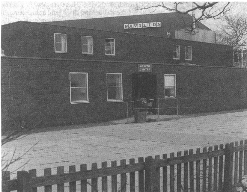
Thornaby Health Centre, Teesside, Cleveland
